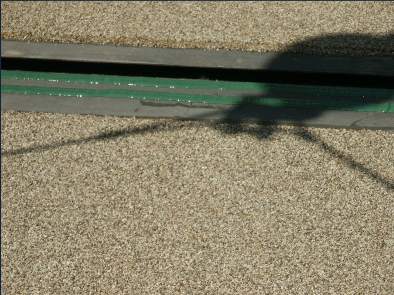
FRP Deck Modules being bonded together
