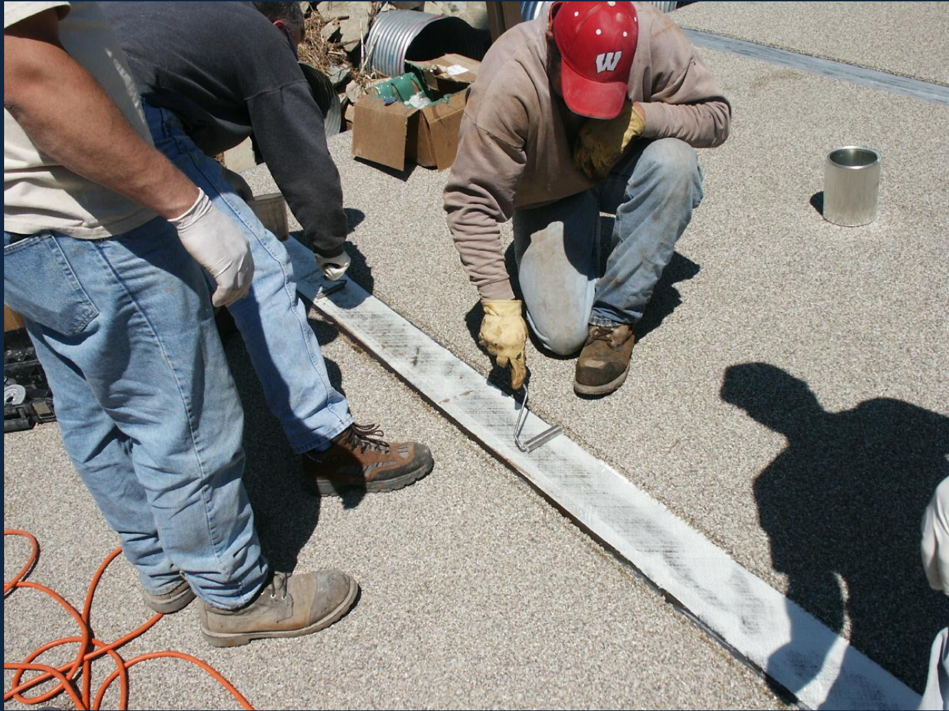
FRP Deck Joints Reinforced with Glass Fabric and Resin
