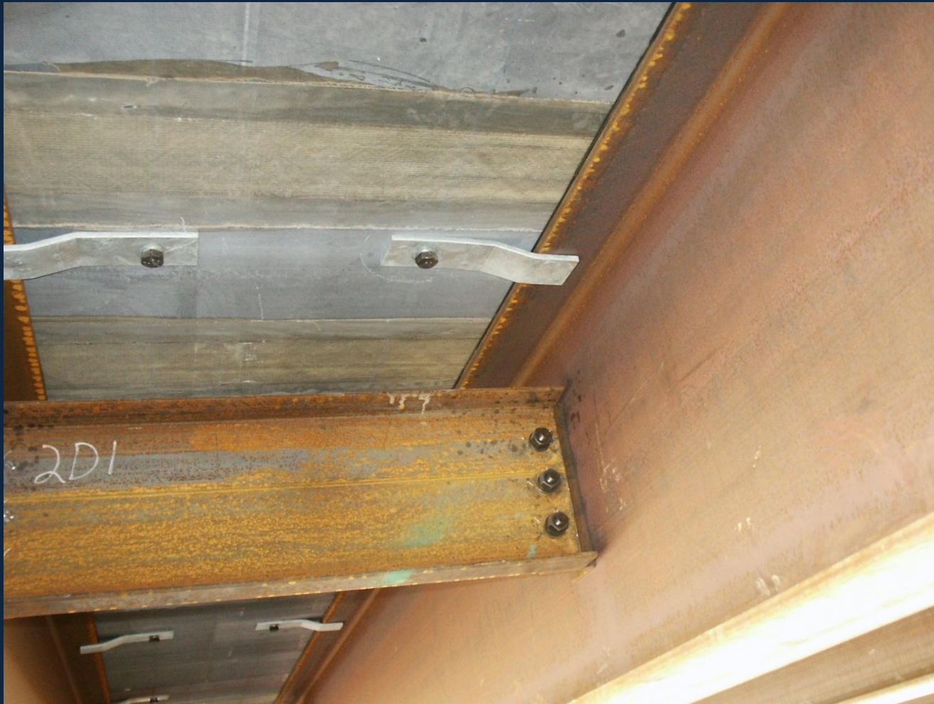
FRP Deck Modules connected to Girders using Spring Clips
