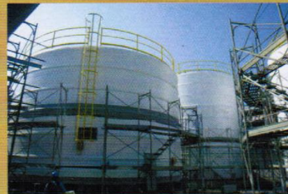
Lifting to foundation & erection
