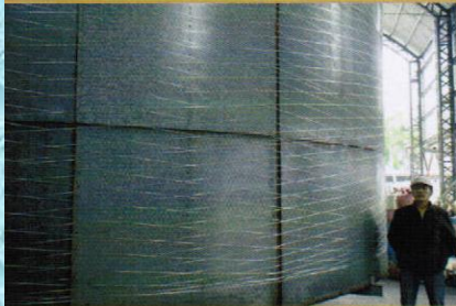
Steel mold prepared & fixed.
