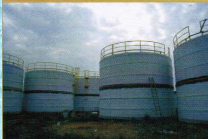
On site pre-assembly before shiping.
