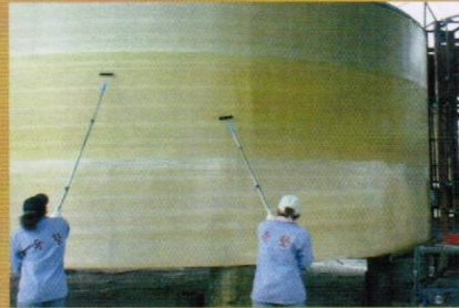
Corrosion barrier, 3mmt applied.
